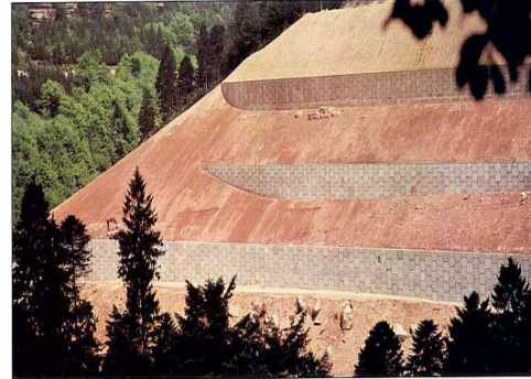
Figure I.27: Renforcement d'un talus
