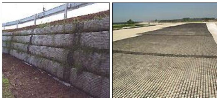
Figure 1.10 Renforcement de sol.
