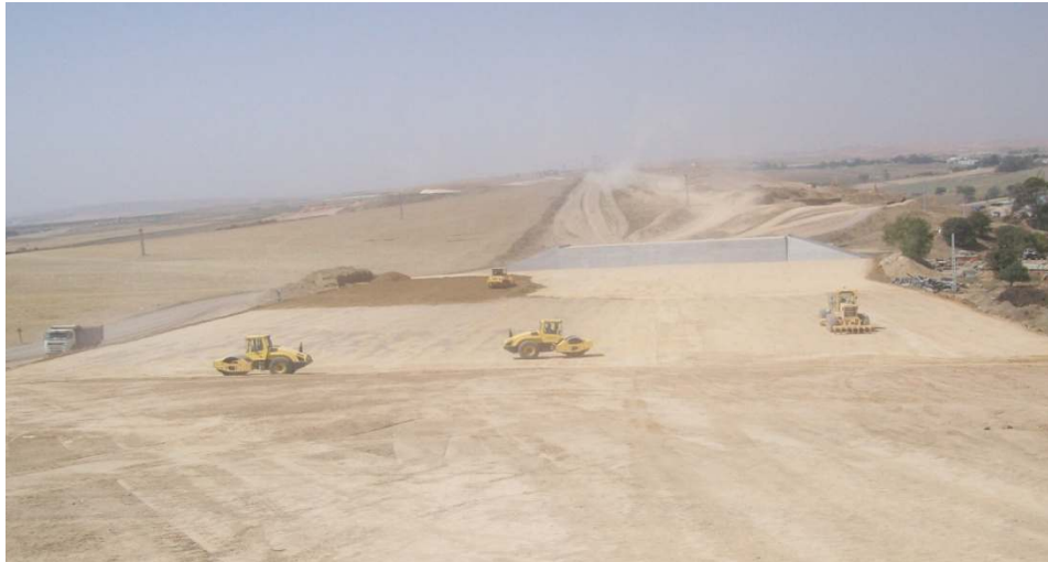
Photo A.4 : section remblai constantine, comp3
