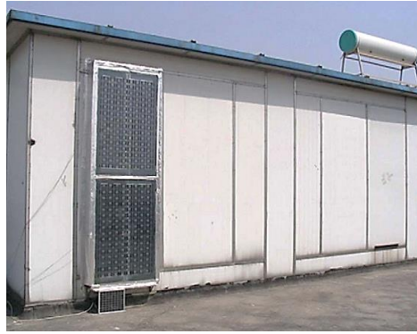
Figure II.10 Image d'un mur Trombe Photovoltaïque [30].
