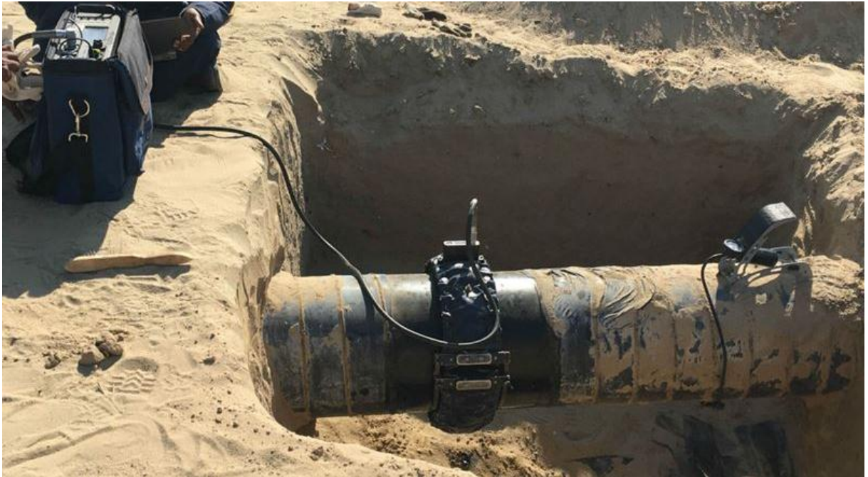
Figure 1.4: Pipeline inspection using guided wave testing (GWT)
