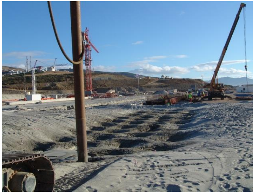
Figure I.2 Processus de vibro-Compactage
