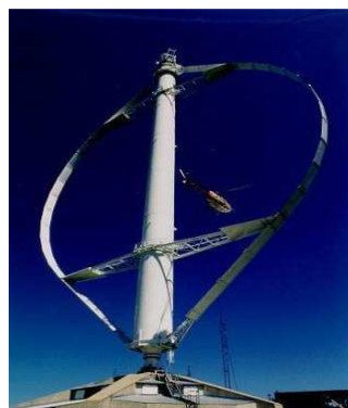
Figure 1.8: Eolienne de Darrieus [8]
